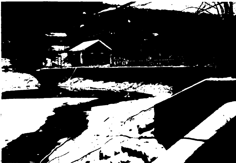
VIEW OF UPSTREAM FACE OF DAM FROM CONTROL OUTLET. HIGHWAY CAN BE SEEN IN BACKGROUND AT LEFT; NOTE LACK OF FREEBOARD OVER TOP OF DAM.
