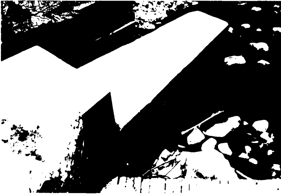
CONCRETE WING WALL ADJACENT TO TAIL RACE; NOTE CRACKING
