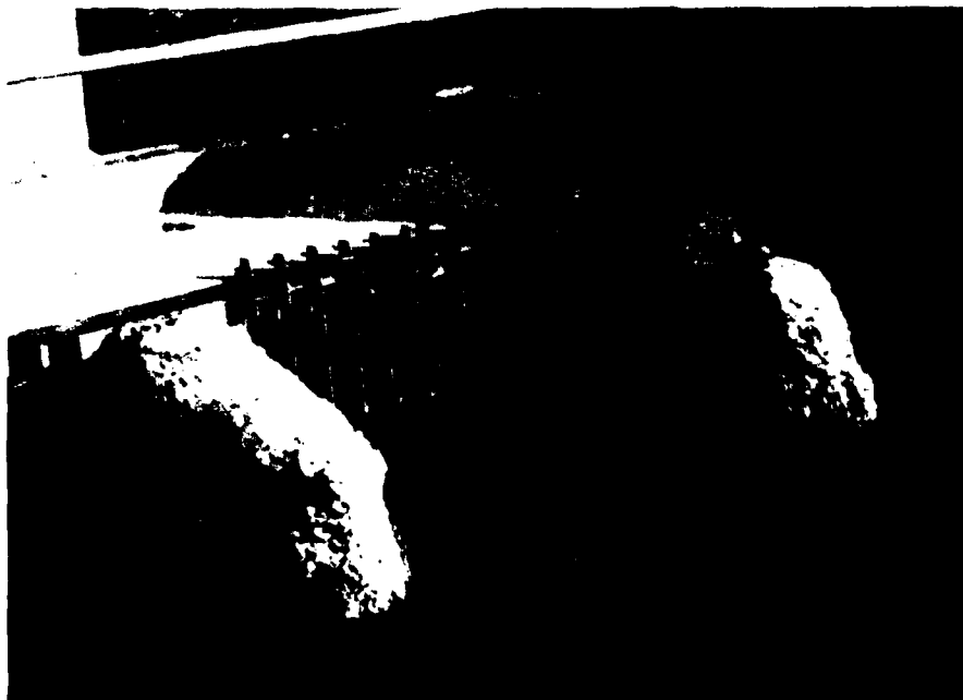
Figure 3 - View of the trash racks and head gates. Note the spalling of the piers.
