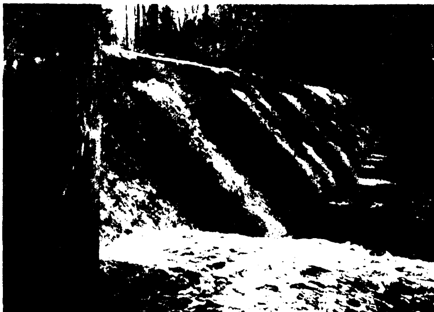
Figure 2 - Looking south along the upstream face of the spillway. Note the erosion at the crest.
