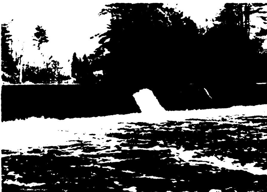
Figure 15 - View of the eroded section of the dam crest.
