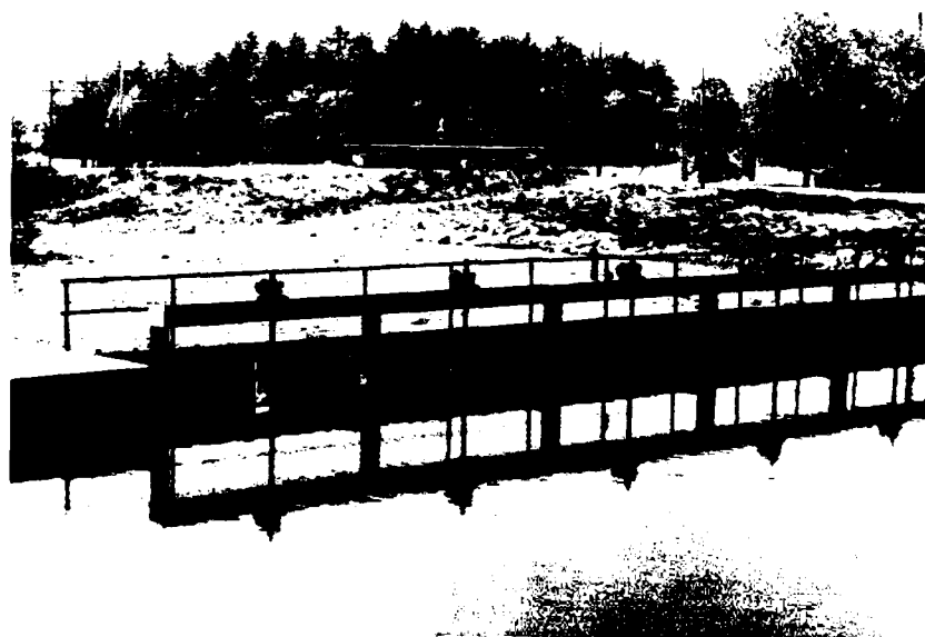
2. View from upstream of operating mechanisms for left side waste gates
