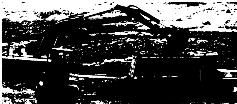
A Warner Swasey Hopto loads unsuitable peat material onto a Mack haul truck. Approximately two feet of peat had to be disposed of. Note water table is right up to ground level.
