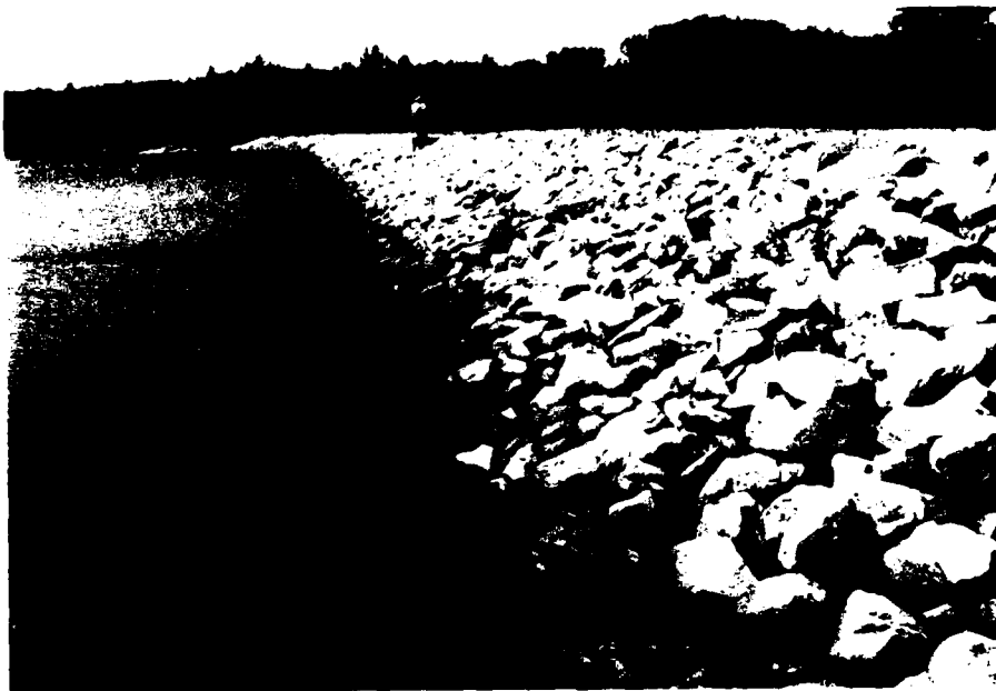
1. UPSTREAM FACE OF DAM SHOWING RIPRAP WAVE PROTECTION AND RESERVOIR DRAIN GATE OPERATOR.
