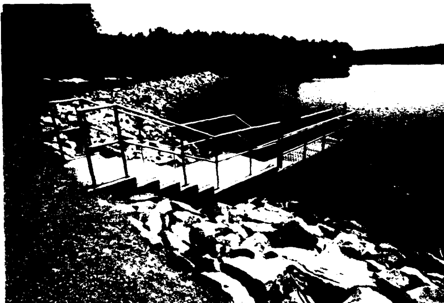
10. FISHWAY INLET STRUCTURE NEAR RIGHT ABUTMENT OF DAM.
