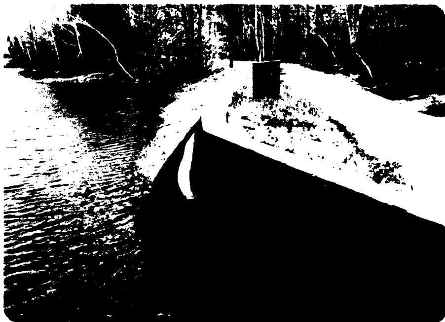
#3. VIEW OF LEFT ABUTMENT AND CORE WALL SHOWING NEW CONCRETE FACING
