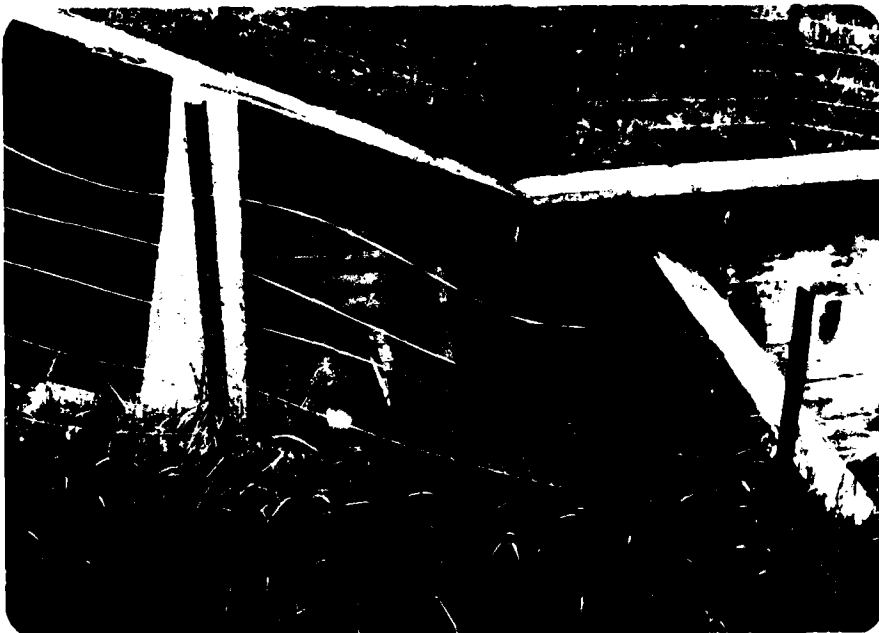
6. Discharge Channel with Cross Beams, Looking East.
