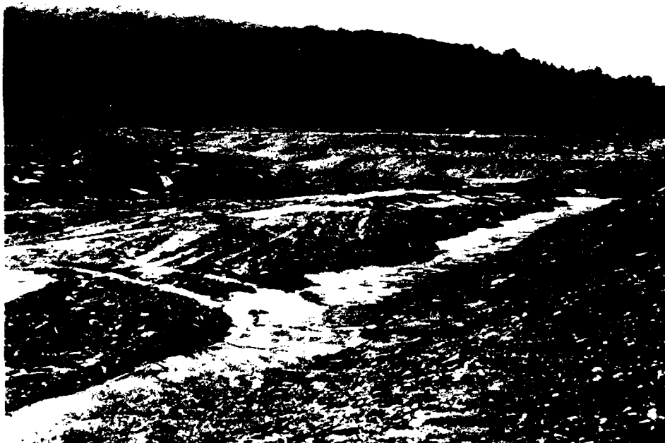
Photograph 2 - View of upstream slope showing riprap and 48-inch riser. Note shelf on upstream slope at approximate elevation 1559 NGVD.
