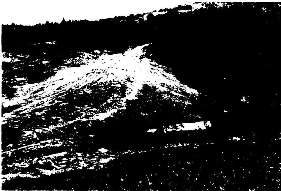
Photograph 1 - Southerly view showing embankment crest and downstream slope. Note standing water and temporary diversion dike at north abutment.
