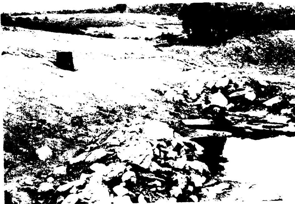
Photograph 3 - View of inlet to 24-inch pond drain at toe of upstream slope and 48-inch diameter riser. Note gully at contact with northerly abutment. Note riprap blanket at normal pool level.
