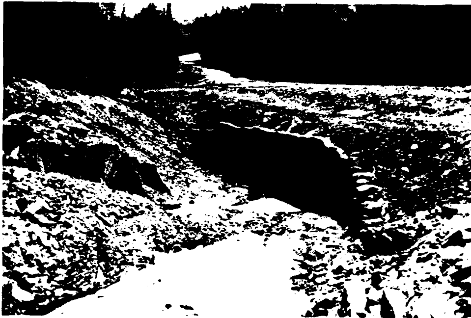
Photograph 9 - Inlet for emergency spillway showing rough and irregular concrete headwall. Note rock in approach channel.
