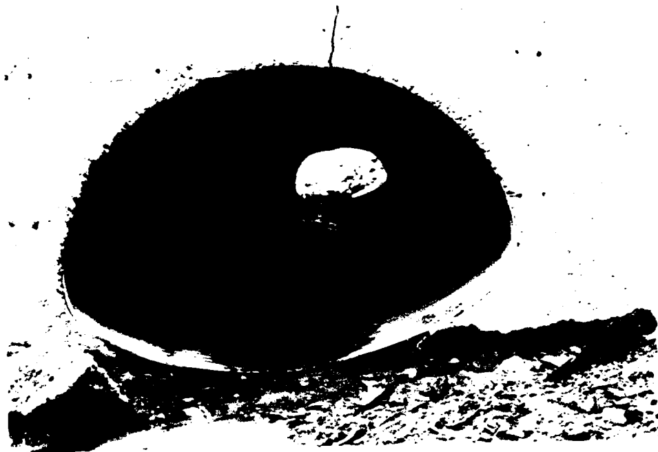
Photograph 11 - Close up of one of three 44" x 72" CMP arch culverts which make up emergency spillway. Note deformation in top of culvert and crack in concrete endwall. Concrete does not surround pipe at bottom.
