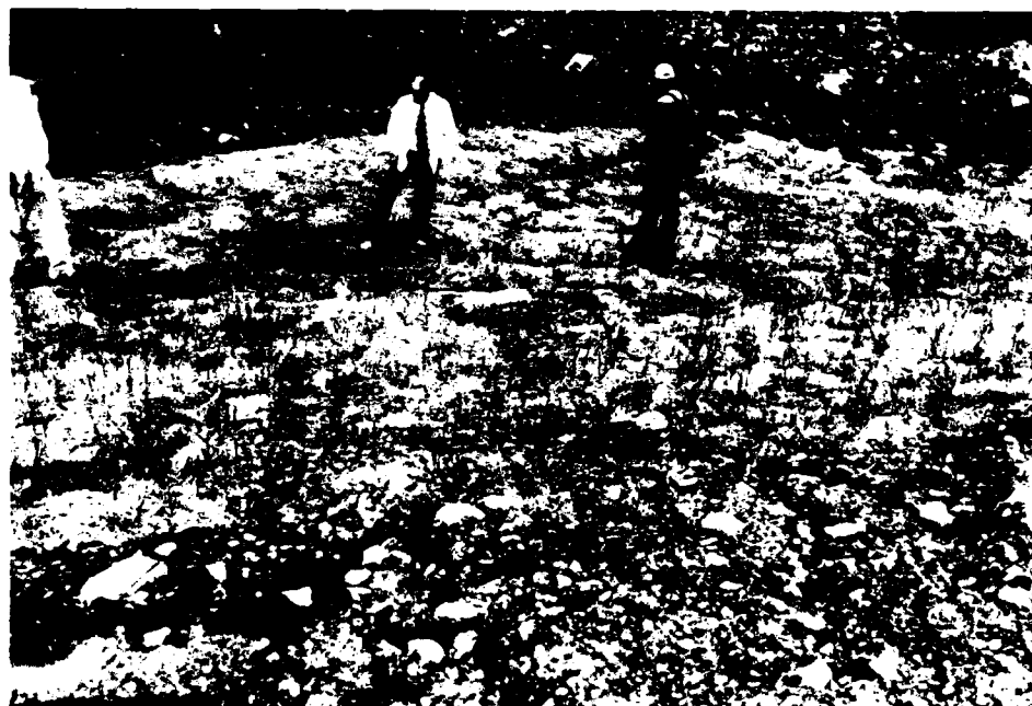
Photograph 6 - View of 3' x 10' area with quick condition at southerly downstream toe.
