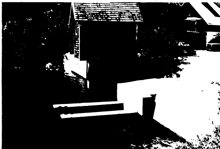
#5 SPILLWAY, DROP-INLET AND GATEHOUSE
