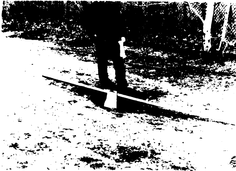
3. View of sinkhole at mid-length of dam crest.
