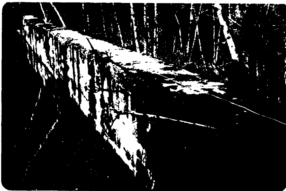
(9) Concrete Dike Upstream of Dam May 8, 1980
