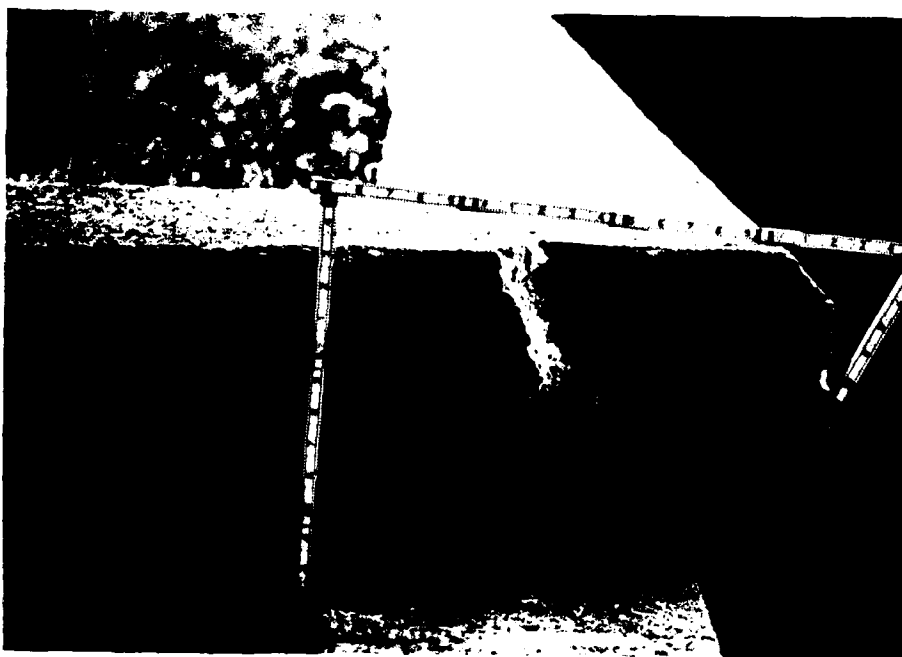
Photo No. 17 - Crack and spalling of upstream end of right training wall of spillway discharge channel.
