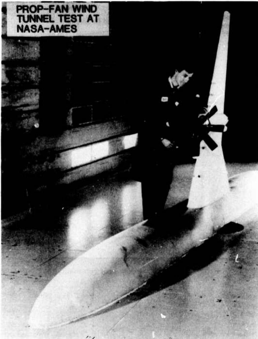
Figure 7. Propfan Mounted on Sweptback Wing in NASA Wind Tunnel
