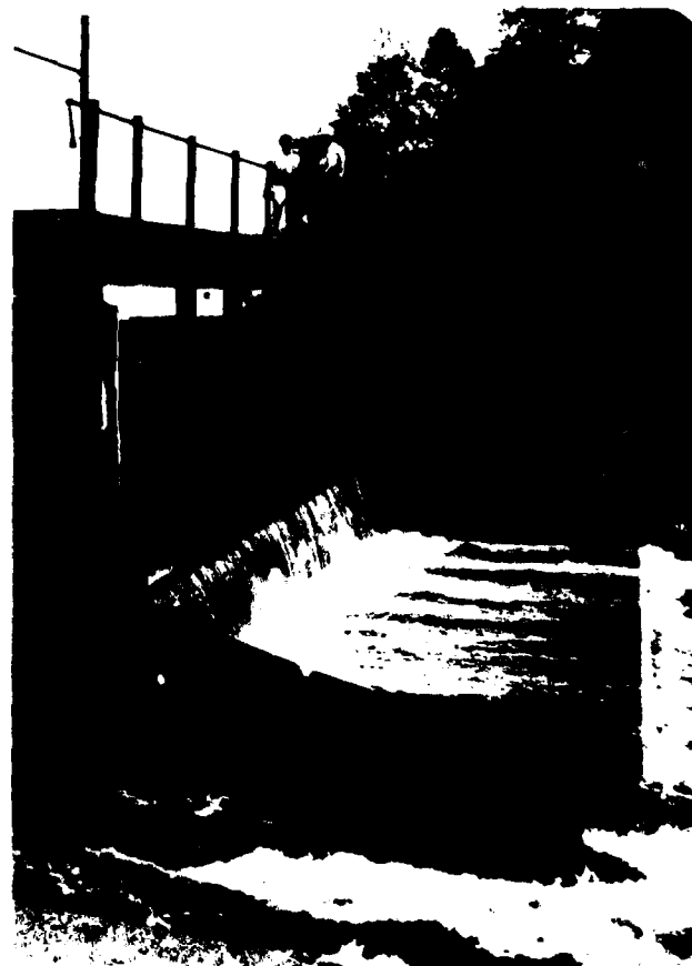
1. Mascoma Lake Dam: Gate House, Stop Log Section and Spillway. Footbridge from Gate House to Spillway.
