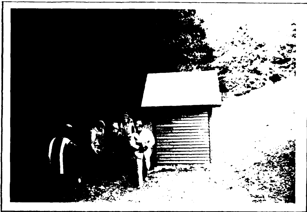
3. GATEHOUSE AT THE DOWNSTREAM TOE OF THE DAM. (12/3/80)
