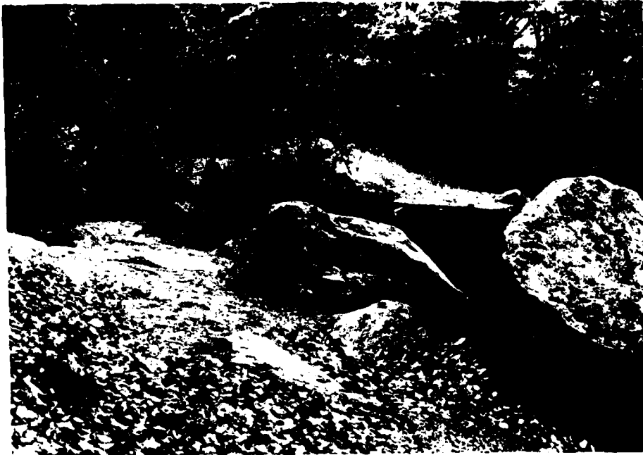
3. Boulders on upstream slope of left dam embankment.
