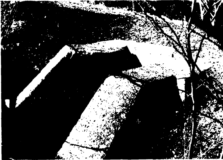
13. Extensive erosion on upstream slope of Dike A at abandoned outlet structure.
