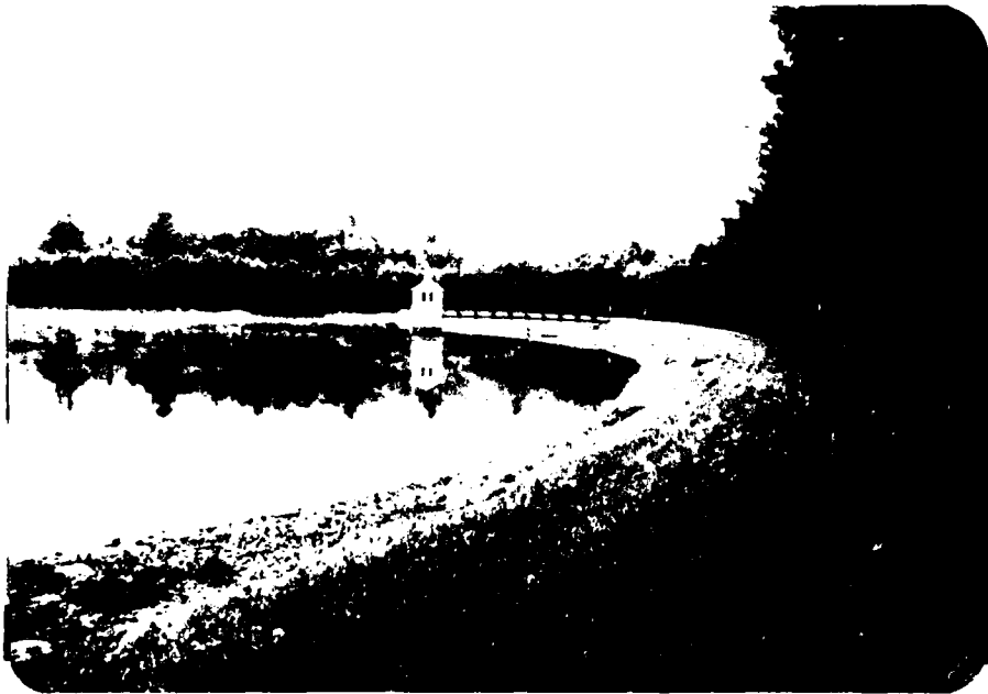
1 VIEW OF DAM FROM EAST END
