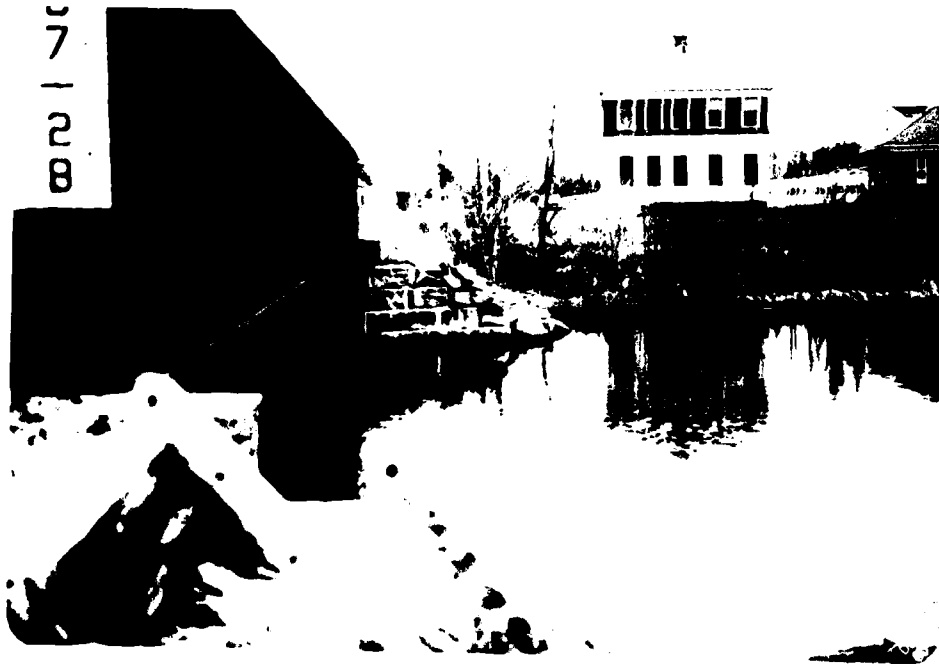
9. Original Riverbed Below Spillway Section of Dam. Abandoned Fishway and Masonry Training Wall at Right, Remains of Wastegate Section of Former Dam at Left Bank.
