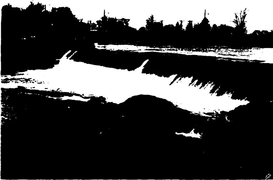
12. Right side of spillway, downstream
