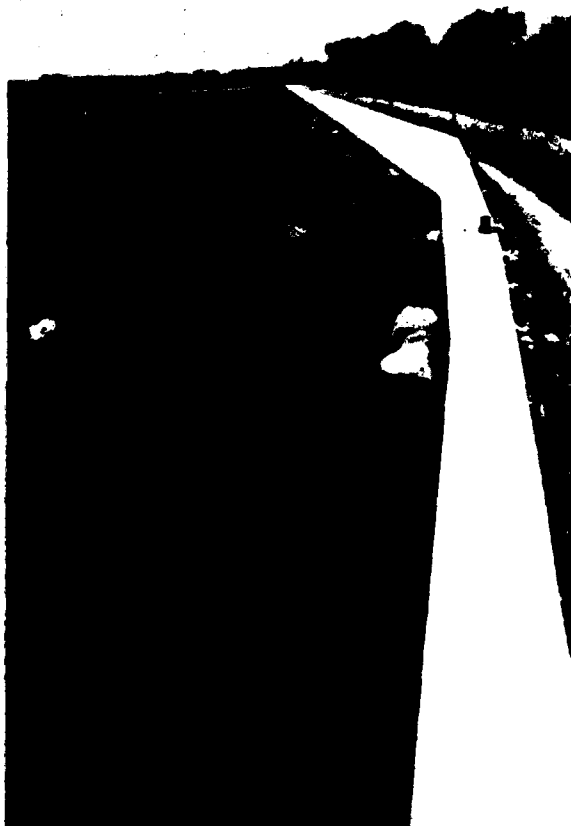
NO. 14 EAST DIKE — UPSTREAM FACE NEAR BEND IN EMBANKMENT WHERE RIPRAP IS MISSING
