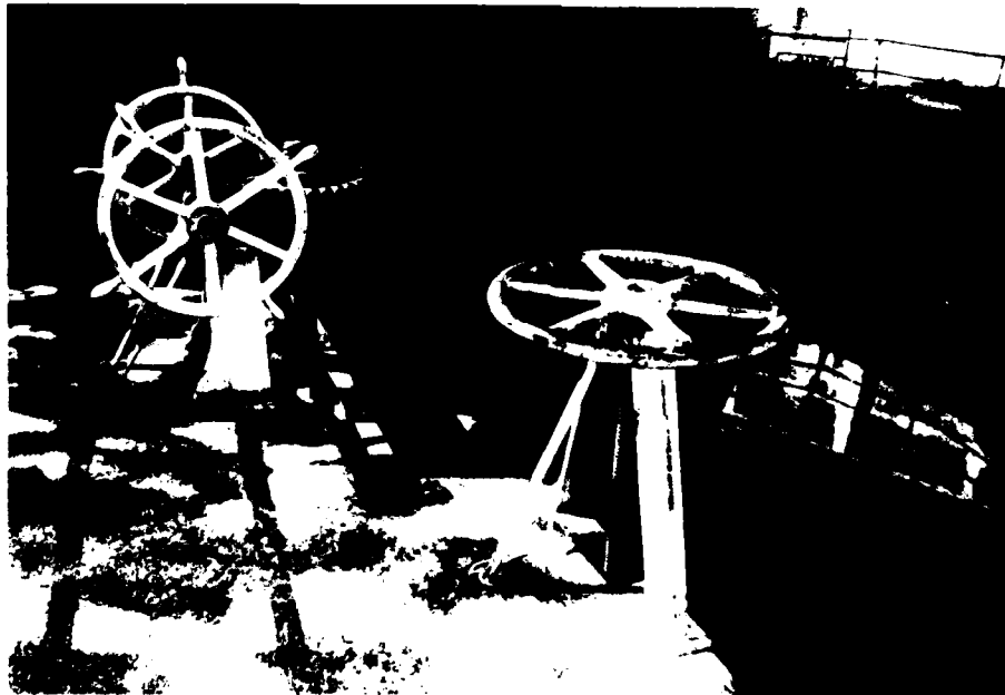
6. GATE OPERATORS ON LEFT ENTRANCE TRAINING WALL OF SCREEN HOUSE.
