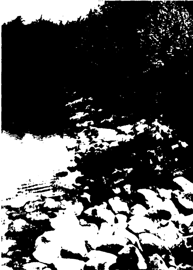
Photo No. 20 Riprap on upstream face from right abutment toward point of curvature.
