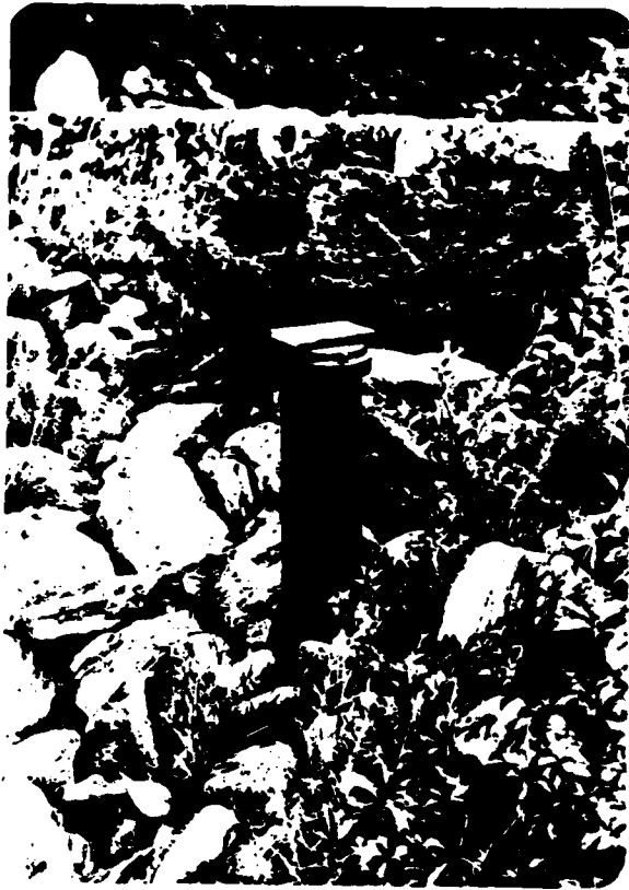
33. Settlement Observation Pipe on Upstream Slope Near Crest of Dike
