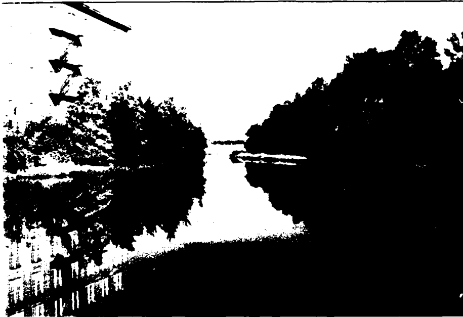
NO. 7 VIEW OF BLACKSTONE RIVER DOWNSTREAM OF SPILLWAY
