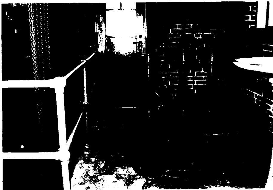
PHOTO NO. 9 VIEW OF OPERATORS INSIDE GATE HOUSE - NOTE CHAINFALL FOR LIFTING SCREENS AND ACCESS OPENING TO WELL
