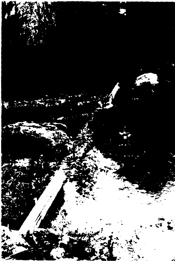
PHOTO NO. 7 VIEW OF EMERGENCY SPILLWAY - NOTE FLASHBOARDS REMOVED OVER APPROXIMATELY 50% OF LENGTH
