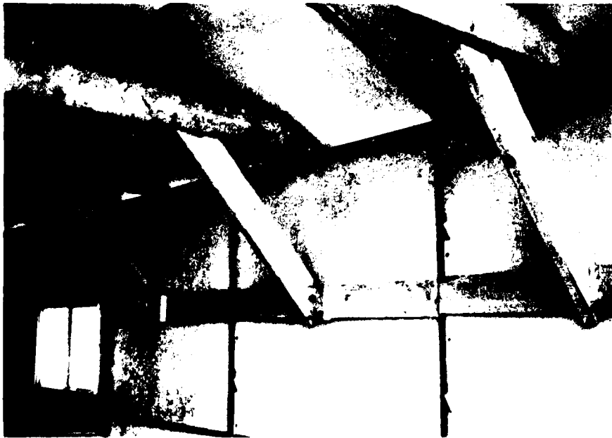
Figure 22. Wood kneebrace system
