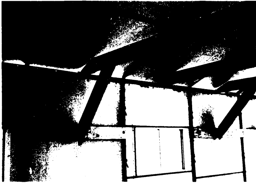
Figure 23. Wood kneebrace attachment to chords and sidewalls.
