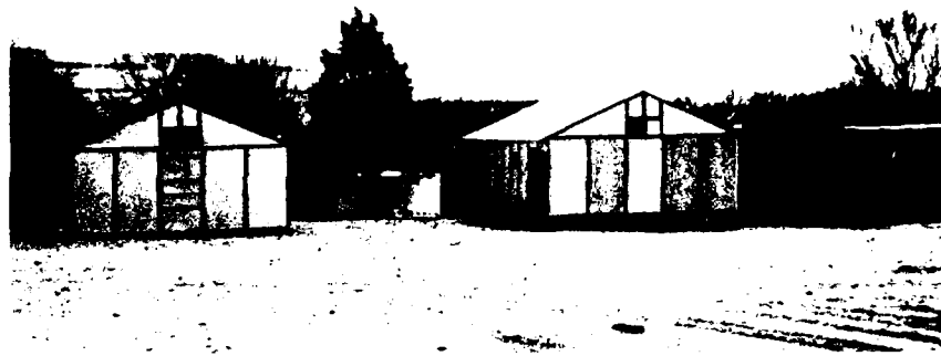
Figure 4. Test structure and control structure on elevated wood baseplates.
