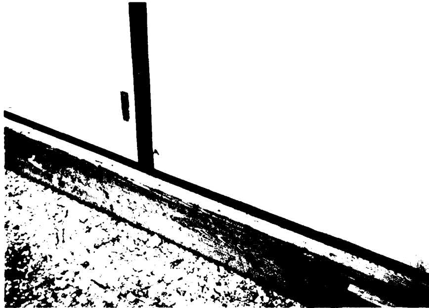
Figure 27. Sidewall moisture damage at panel base.
