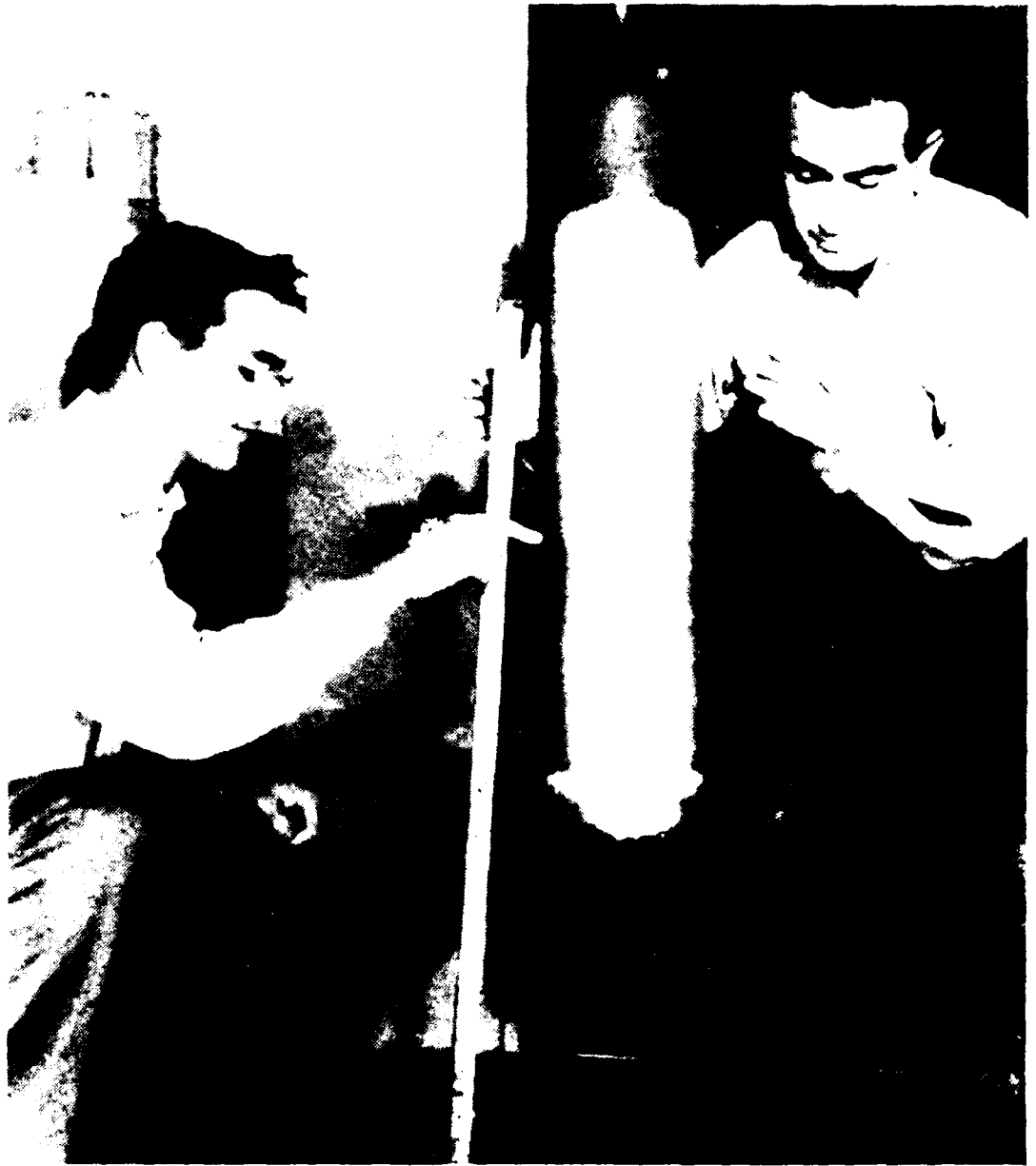
Dr. Talbot A. Chubb (left) and Dr. Herbert Friedman shock testing a Deacon rocket payload.
