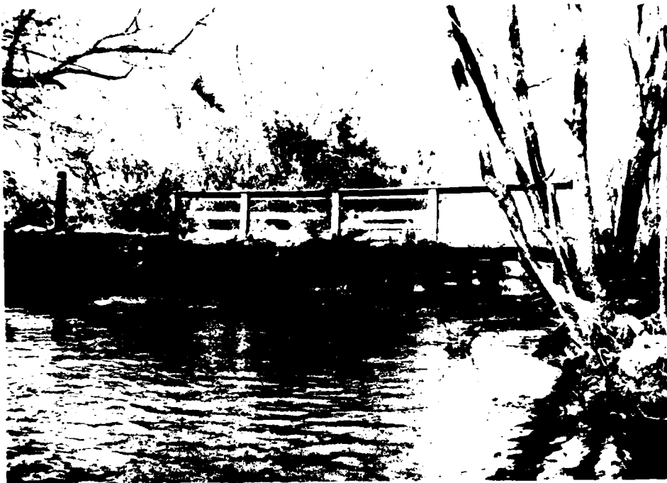
C. Leith Creek – Just below McKay Street, looking upstream.
