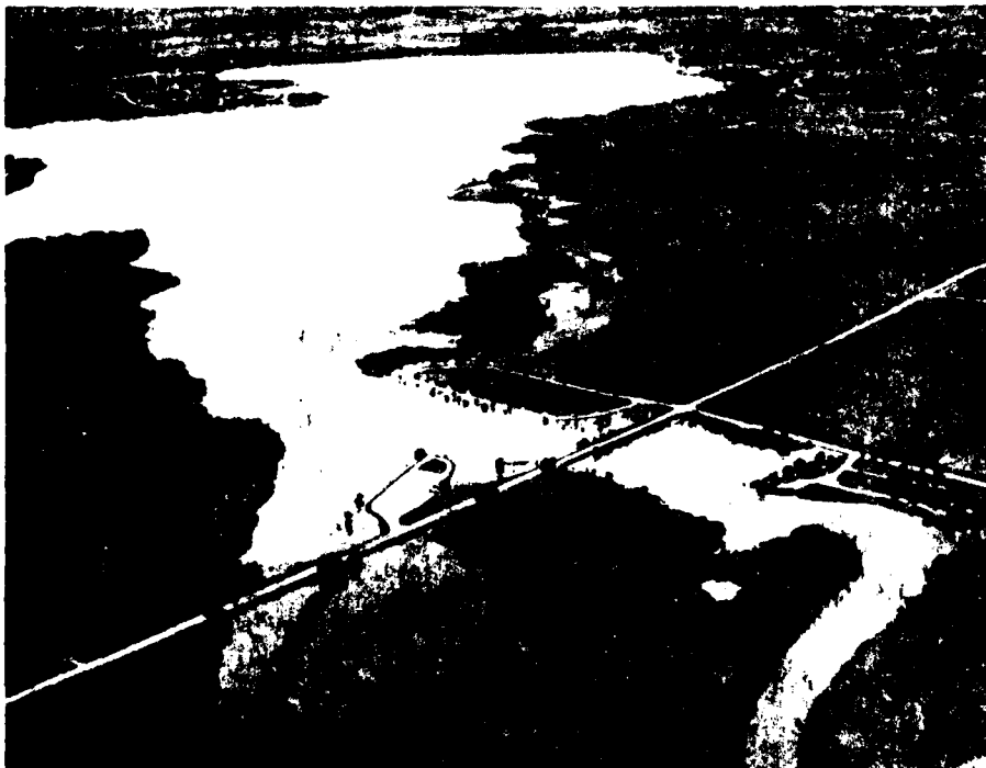
Figure 10. View of Salt Creek Dam No. 14 - Pawnee Lake, 13 June 1984. (Pool Elevation - 1246.8 feet m.s.l.)
