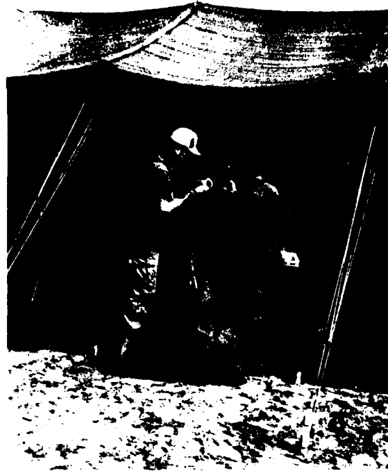
Figure 60. Becketing the vestibule to the extender
