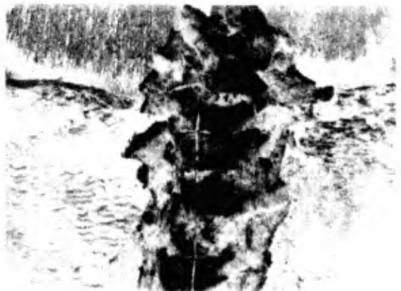
Fig. A.2.5—Exudation and incrustation
