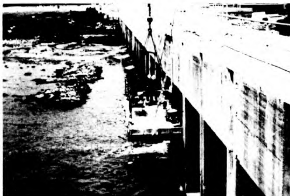
Figure 30. Crane supporting horizontal drilling operation, Starved Rock Lock and Dam, Illinois Waterway
