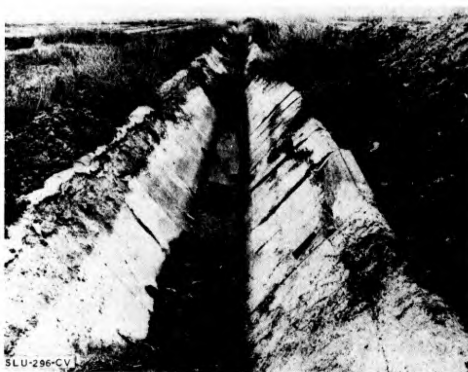
Figure 8. Concrete-lined ditch approximately 1 mile north of Delta-Mendota Canal, California. Concrete containing Type I cement was placed in 1957 and photographed in 1962 (after Bellport 1968)
