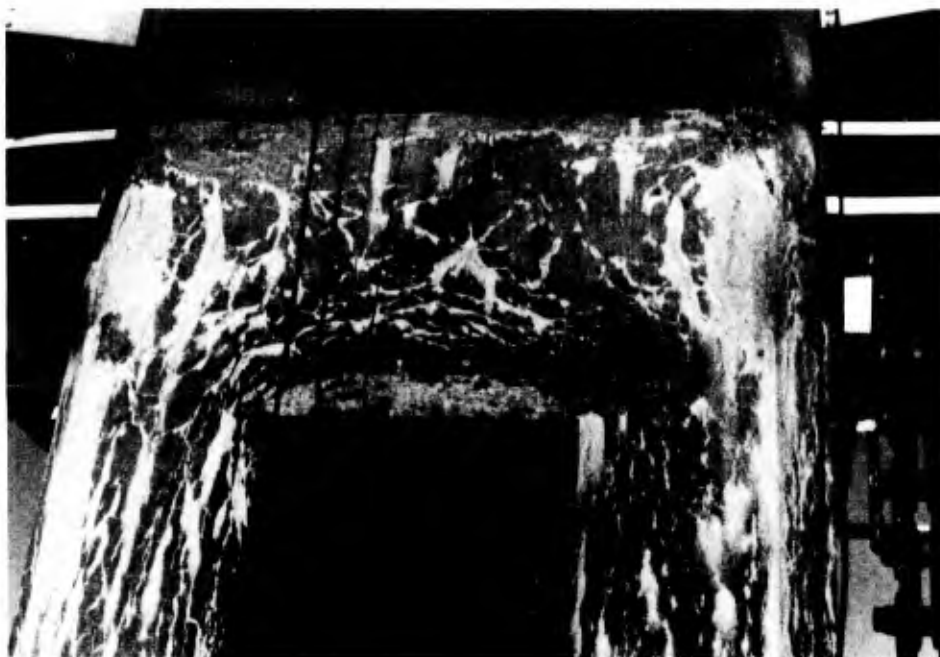
Figure 11. Service bridge support columns, Lock and Dam No. 24, Mississippi River; alkali-silica reaction product present at cracks
