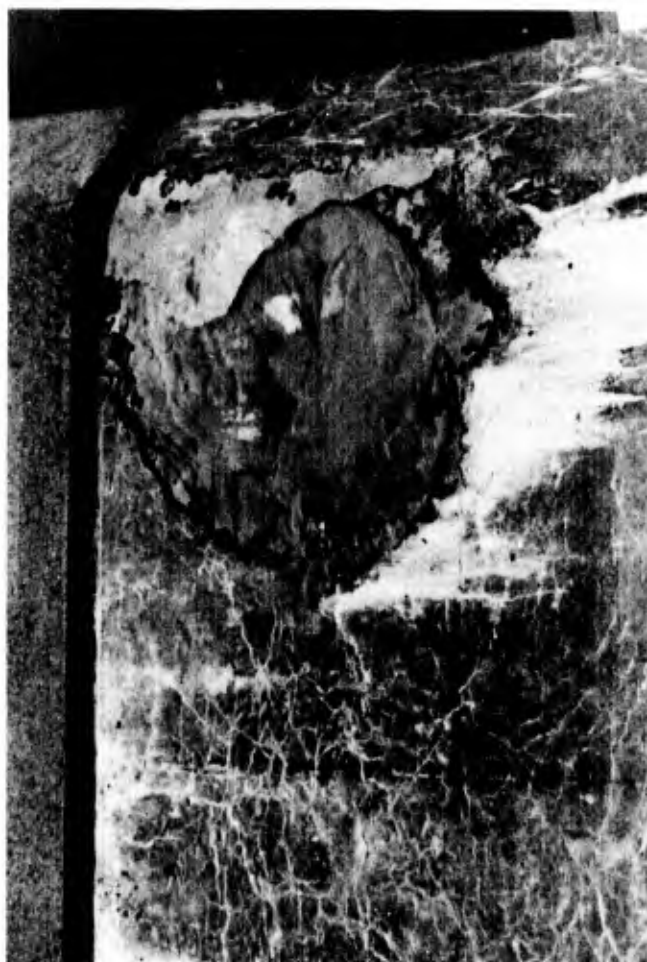
Figure 16. Poor repair; cement mortar repair with an overlay of epoxy. Overlay has failed and exudation coming from beneath the cement mortar repair. Lock and Dam No. 24, Mississippi River
