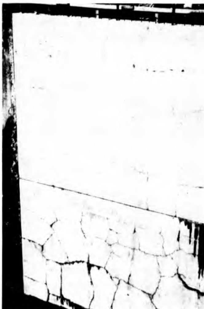
Figure 6. Thermal cracking in lock wall resurfacing concrete
