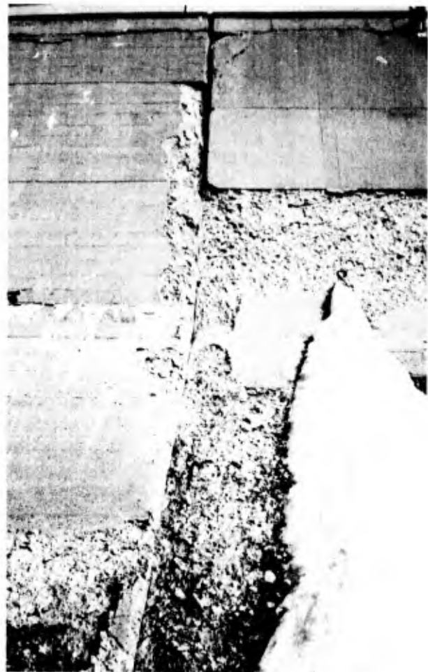
b. Ice formed from water coming out of form tie hole
