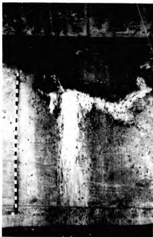
Fig. A.1.1.g—Random cracks (wide)
