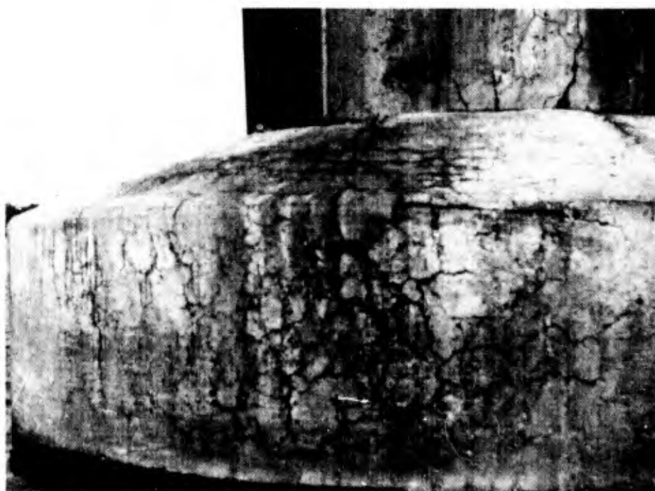
Figure 10. Expansive cracking in pier pedestal due to alkali-carbonate rock reaction
