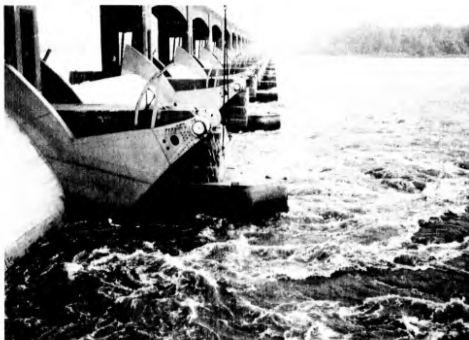
Figure 20. Piers at Lock and Dam No. 24, Mississippi River, with wooden platform in place to facilitate pulse velocity measurement
