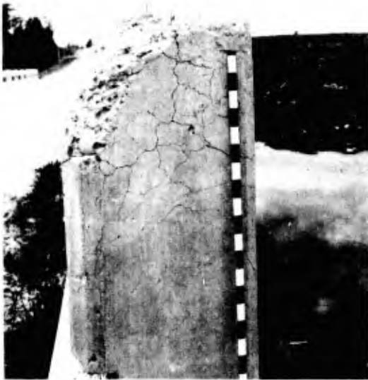
Fig. A.1.2.c—Pattern cracking (wide)
