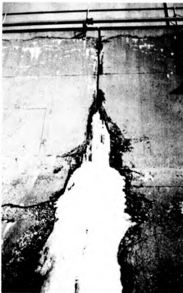
a. Ice over vertical construction joint
