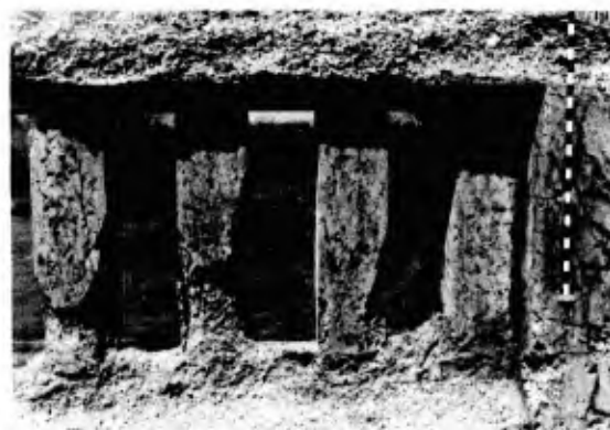
Fig. A.2.9.5.a—Scaling (very severe)
