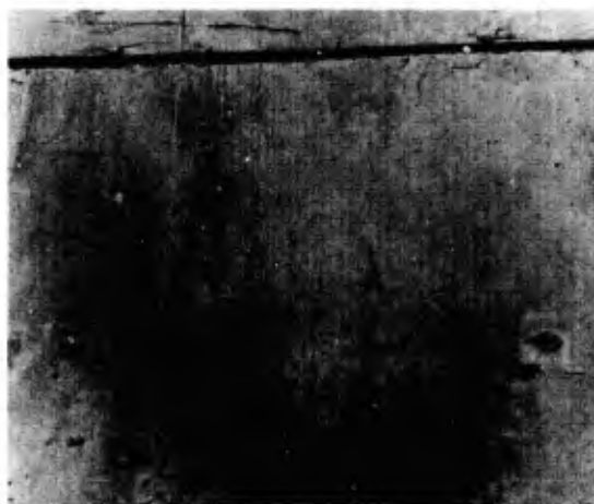
Fig. A.3.2—Sand streaking on a vertical formed surface
