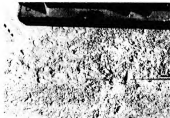
Fig. A.2.9.5.b—Close-up of scaling (very severe)
