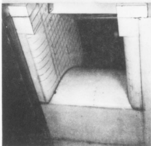
Upstream face of spillway bay without bridge.
