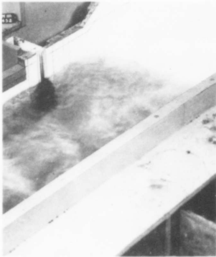
Spillway flow 2,500 cfs.
