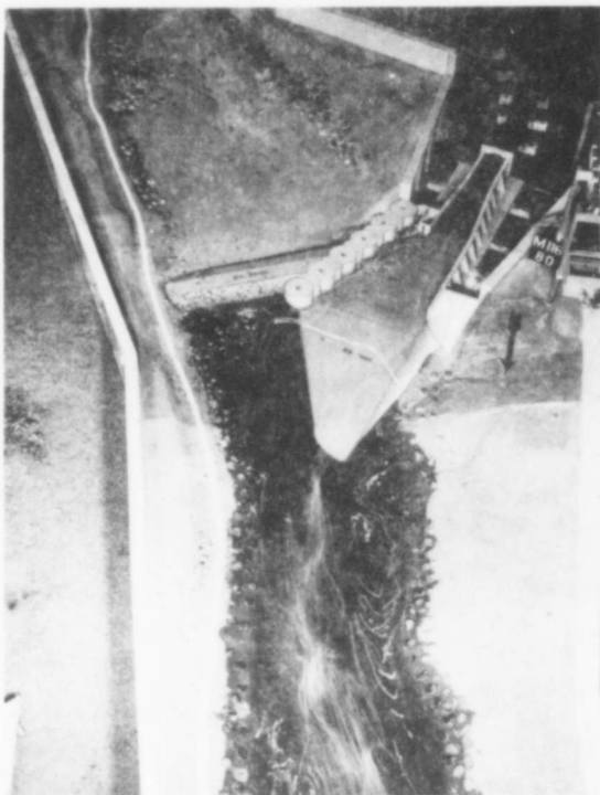
Downstream cofferdam and outlet.
