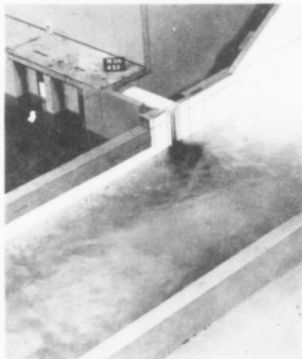
Spillway flow 5,000 cfs.
