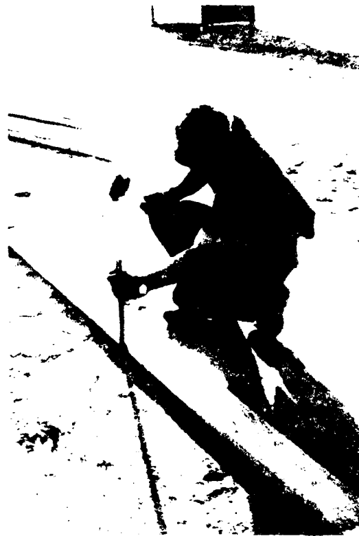
Figure 19. Baseplate stake driving.
