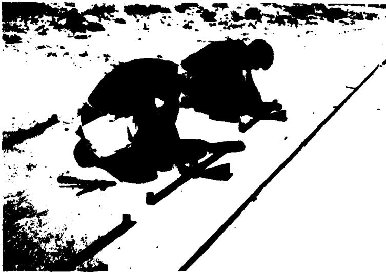
Figure 21. Eave angle assembly.
