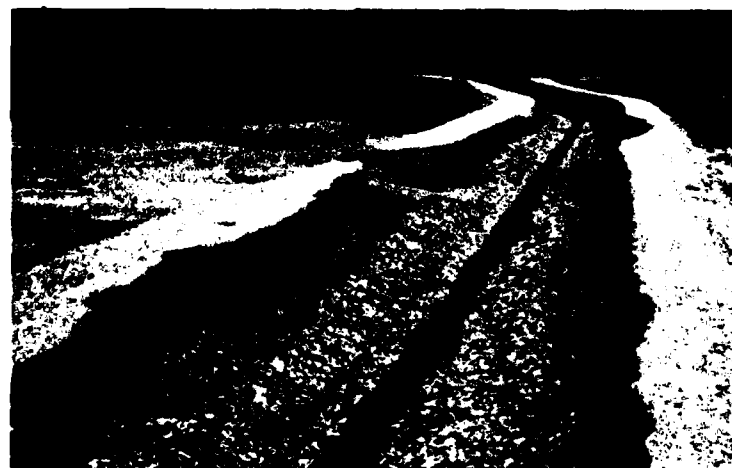
5. A specially constructed narrow, deep channel to carry low winter flows. The narrow channel is formed by rock-filled wire gabions.
