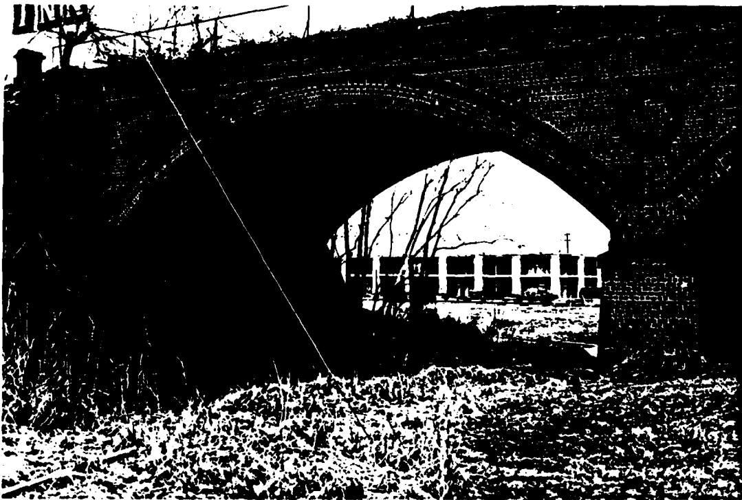
Figure 12b. South side of brick arch viaduct 400 feet north of Louisville Road; constructed 1859.
