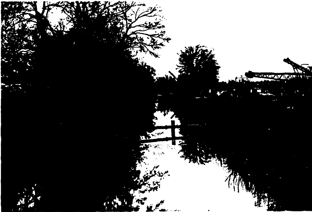
Figure 14a. View north along Springfield Canal from Gwinett Street.
