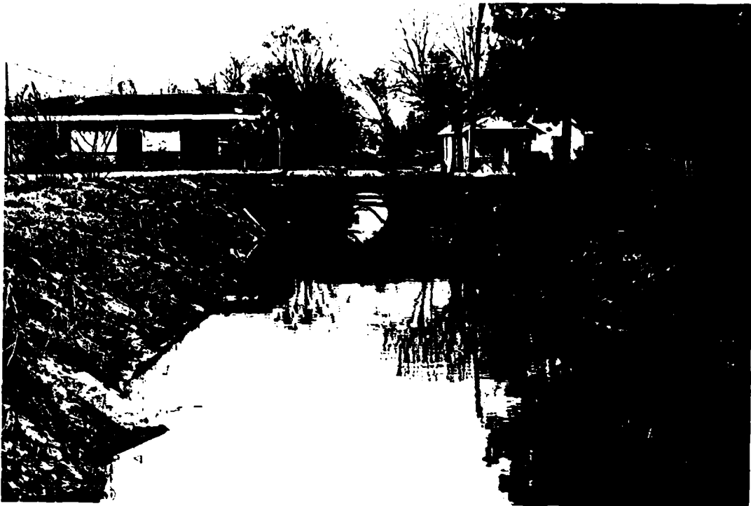
Figure 15a. Ogeechee Road bridge as seen from Victory Drive.
