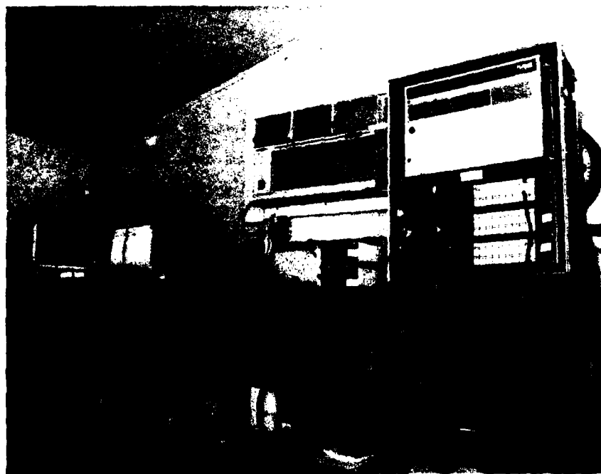
b. Instrumentation room.
