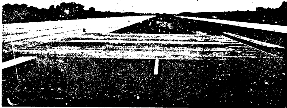
FIG. 4 SINGLE AM-2 MAT ON THE RUNWAY
