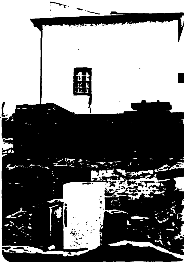
House Moved and Raised
