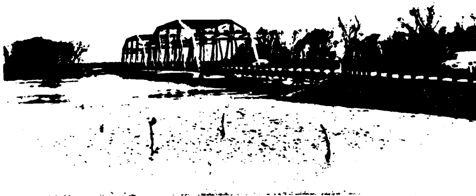
Upstream of Minnesota Highway 1 Bridge looking west, Oslo, Minnesota (taken 8 April 1978).
