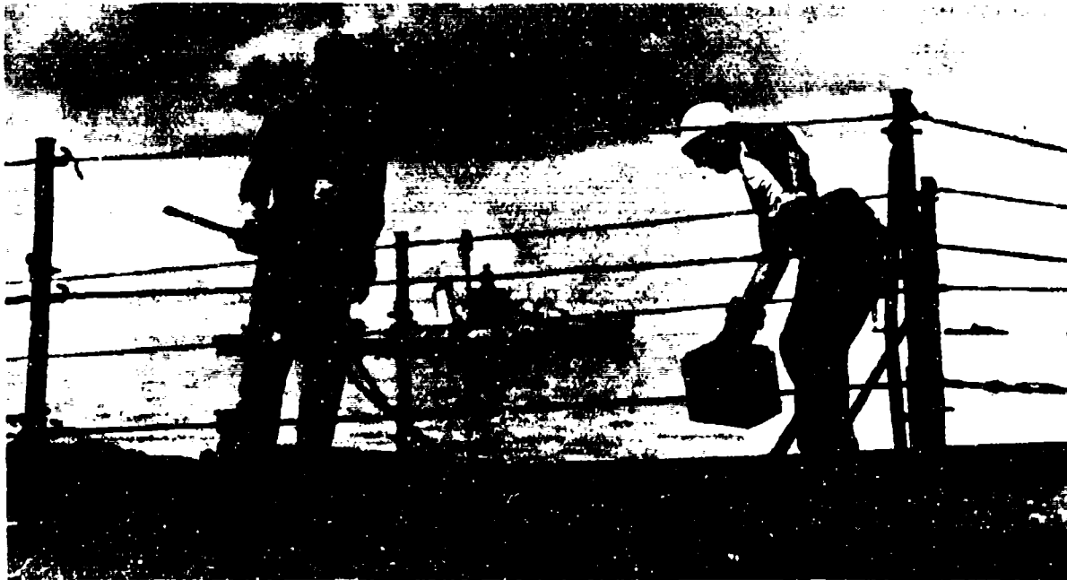
Figure 32. Welder aboard USS Hughes (DD-410) during preparations for towing it after CROSSROADS .
