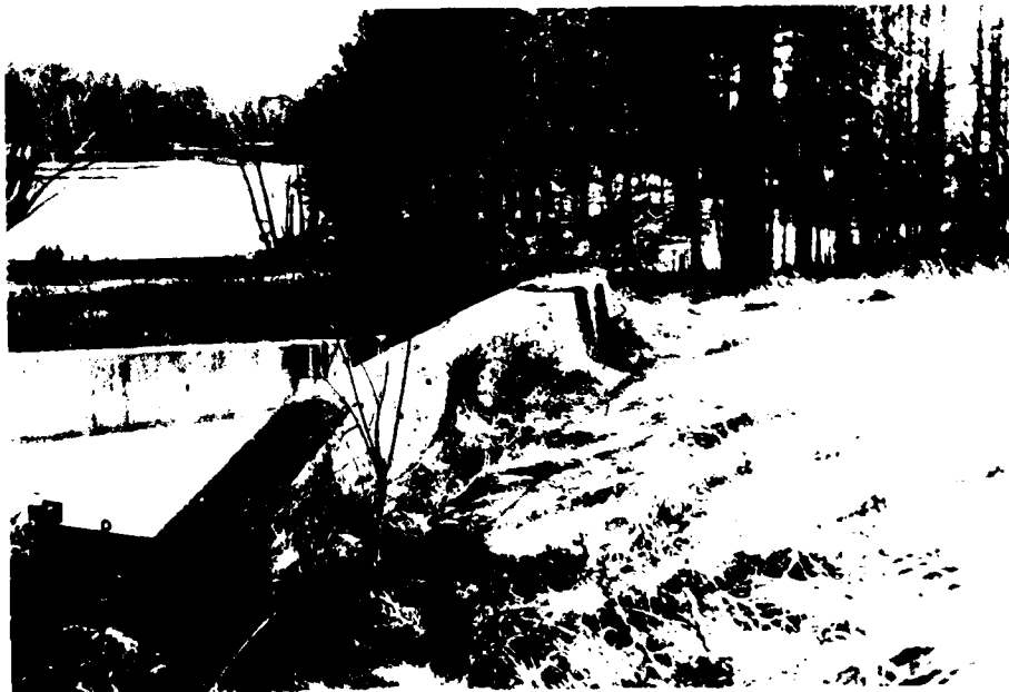
Photograph 12 - Typical low area behind spillway walls. Areas are approximately 1 foot lower than the top of dam. There are no cutoffs or projections of the spillway walls.
