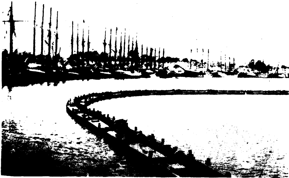
Suction dredge at work in the Inner Harbor, San Pedro, 1902.
