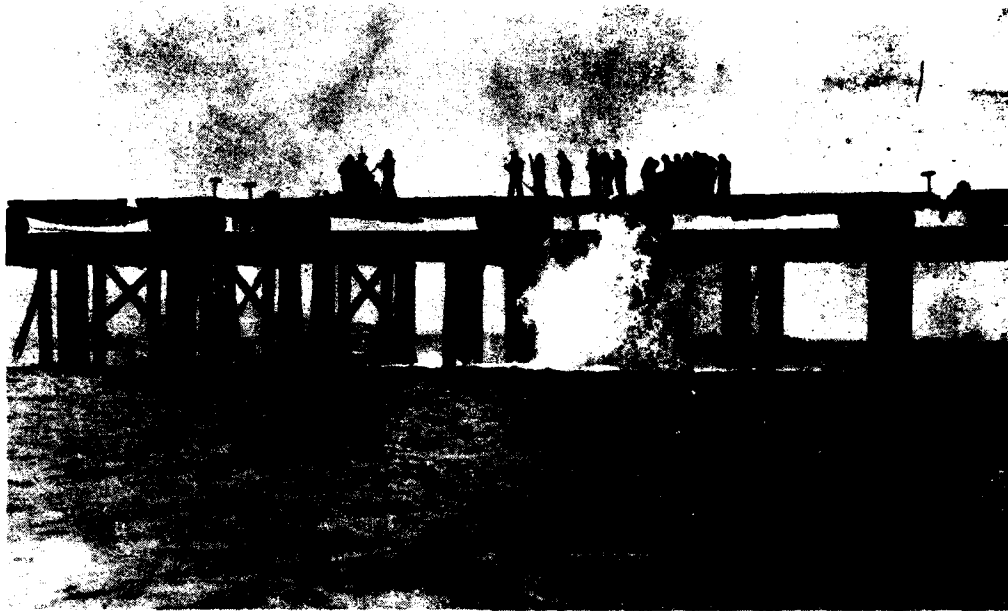
Prying stones from flatcars for the breakwater in 1903.
