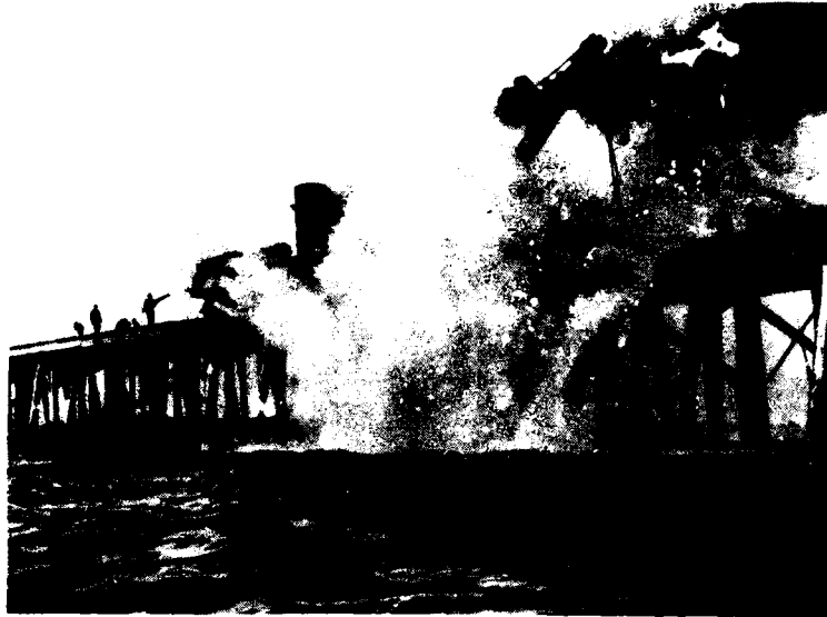
Derrick unloading stones for the superstructure.
