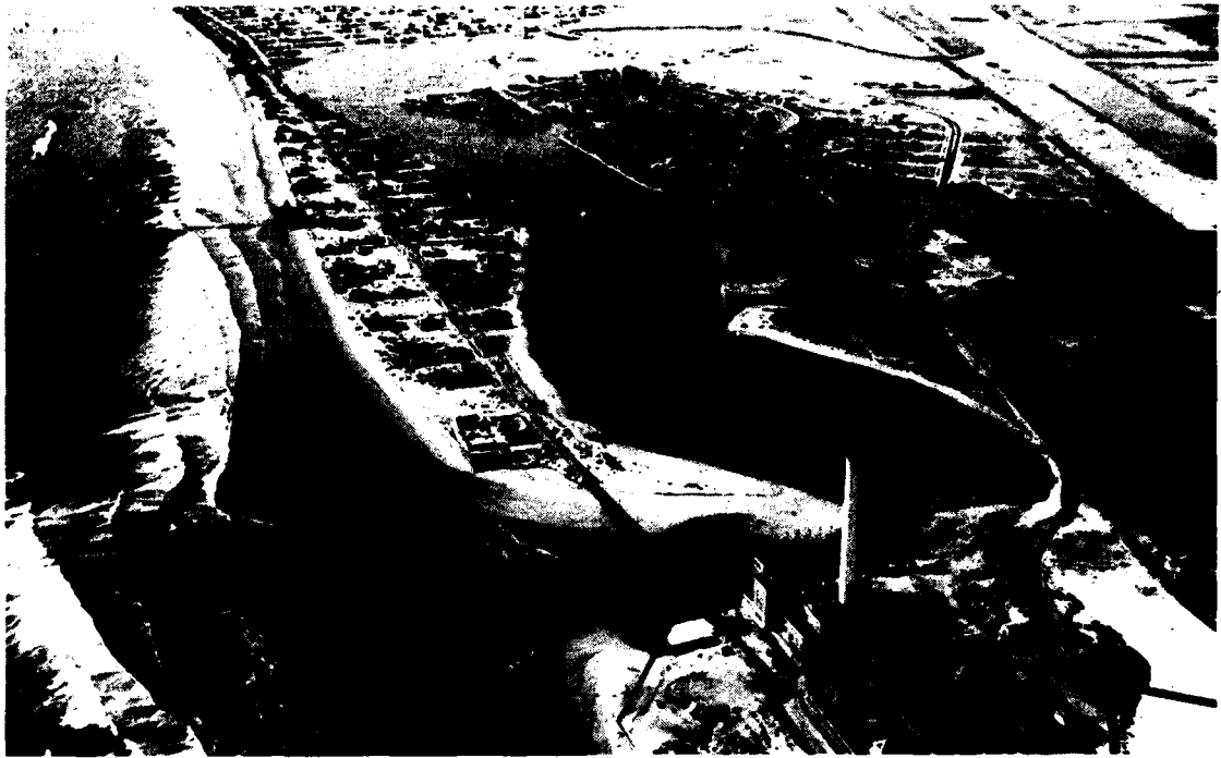
Alamos Bay in 1928. Pacific Electric Railway trestle lies across mouth of the bay.
