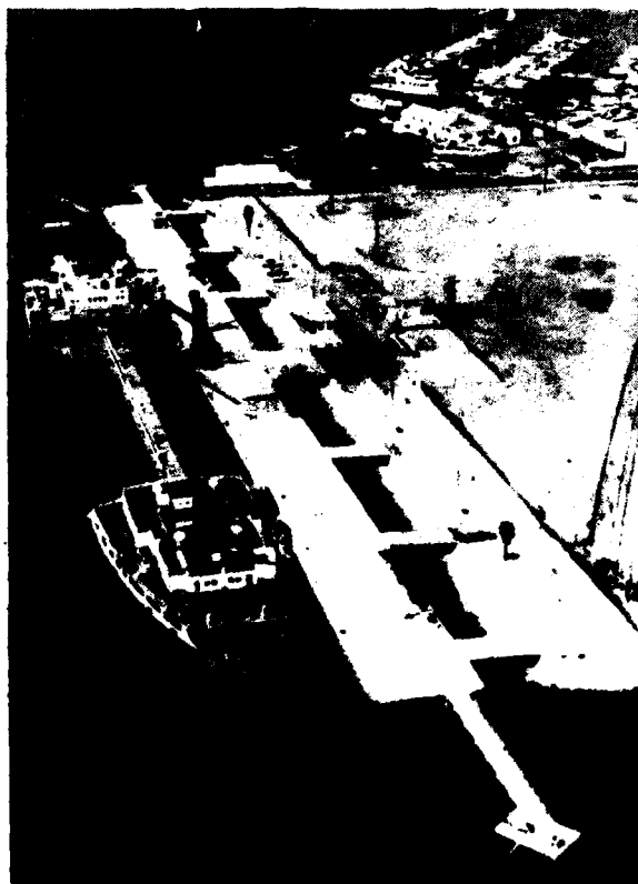
Supertanker terminal at Los Angeles Harbor handles ships carrying 500,000 to 1 million barrels of oil. Pushbutton operated, the facility will unload a ship in a day and a half. The Sansinena , which blew up in the Los Angeles Harbor in December 1976, is shown in this photo at dockside in 1971.
