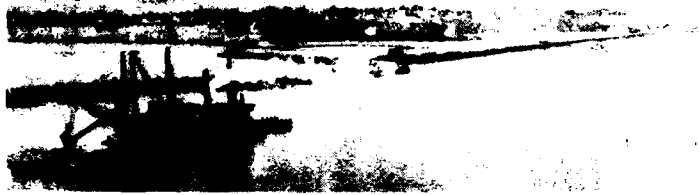
Panorama from Deadman's Island showing dipper dredge at work in channel about 250 feet northward from island in November 1903.
