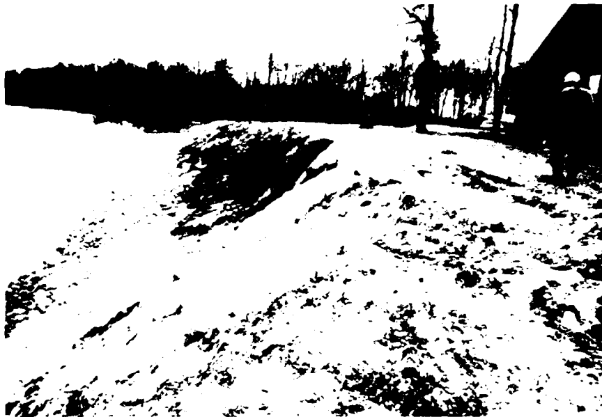
Figure 68. Serious scour occurred on the upper bank in Work Area 6 during the 21 November 1977 storm event, Batupan Bogue (25 January 1978)
