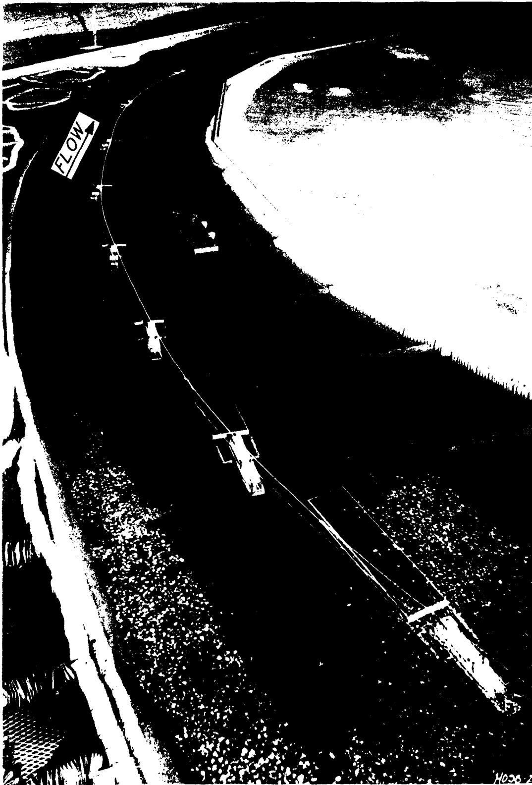
Photo 4. Path of downbound tow passing a tow tied to mooring cells at location 4; discharge 150,000 cfs
