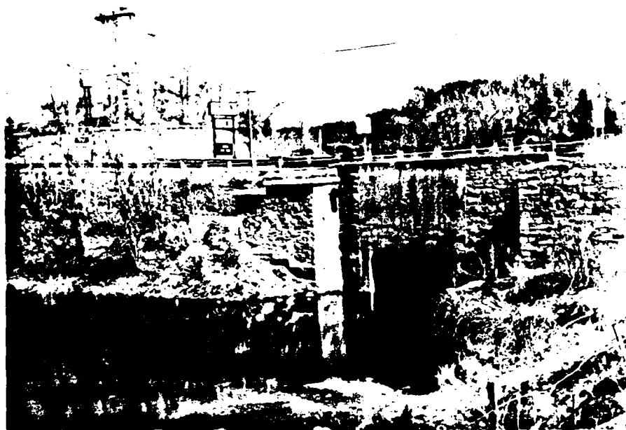
Photo 1. Upstream view of the dam from parking lot at edge of pond. Note cement bag retaining wall at left end of culvert embankment.
