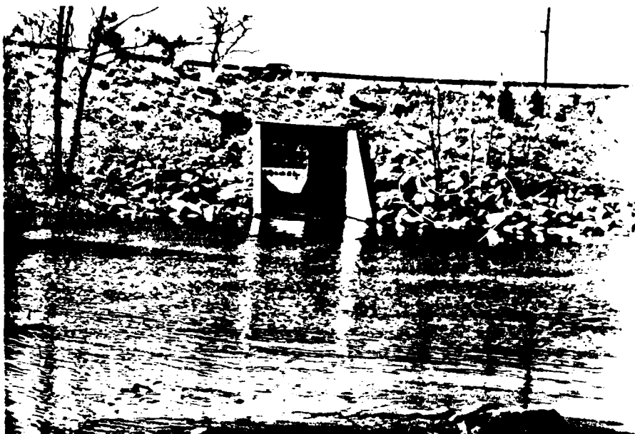
Photo 3. View of downstream slope of dam and spillway weir on upstream side (as viewed through the culvert). Note erosion along both wing walls of culvert outlet.
