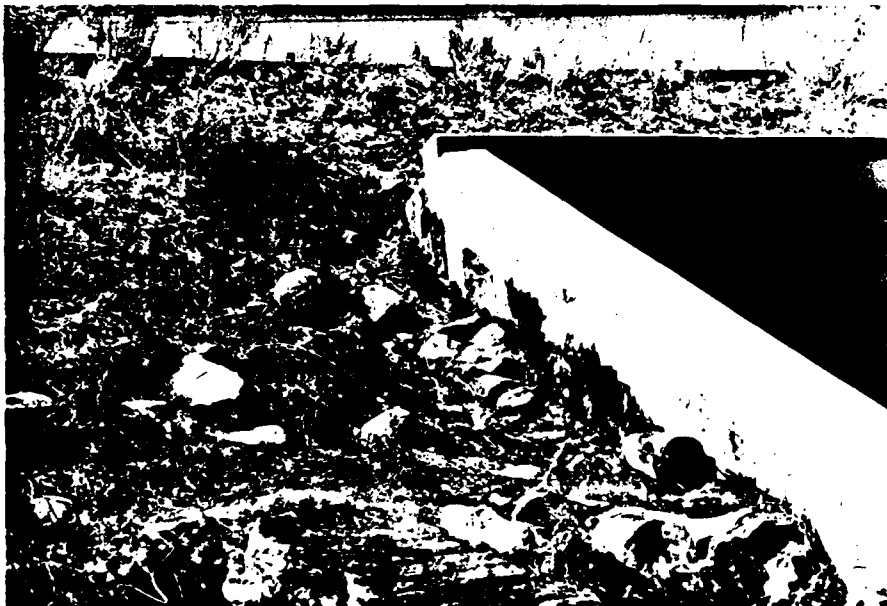
Photo 4. Closeup of erosion along the right wing wall of the culvert outlet.
