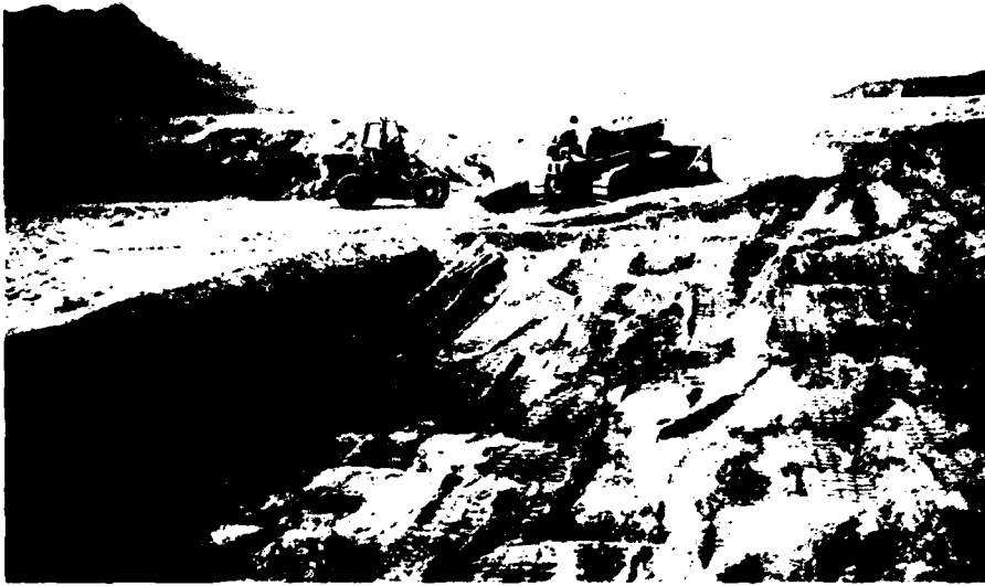
Figure 6. Fill material for eroded levee areas was secured from the channel bed
