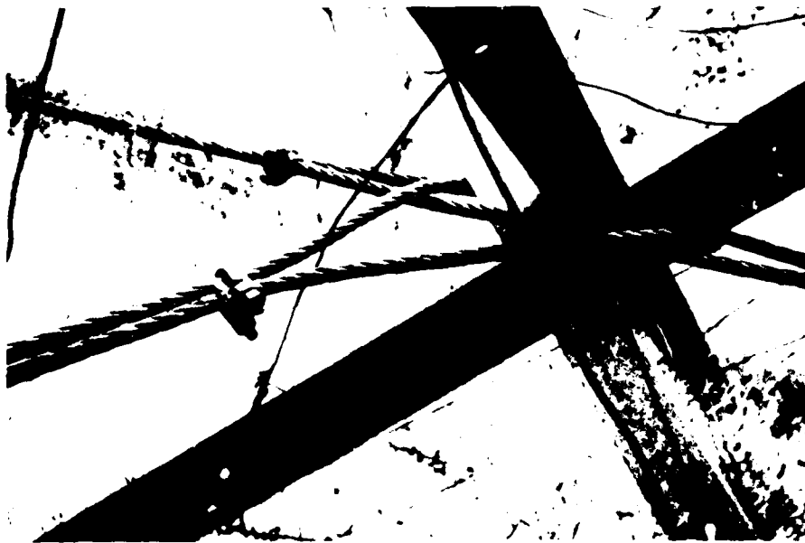
Figure 13. Jacks units are connected with steel cable; this figure shows the cable configuration at the junction of a main-line jetty and retard line
