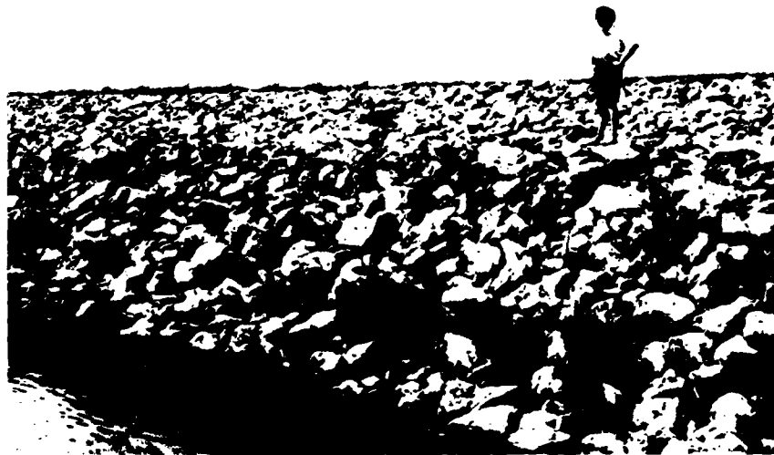
Figure 25. Republic River at Milford Dam Outlet Channel, Kans. Typical view of the revetment toes as seen by the MRD-MRK inspection team in May 1977. The engineer in the photograph is standing on the horizontal blanket at the break in slope between the blanket and the slope to the water. (Source: Reference 11)
