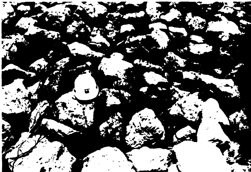
Figure 28. Republican River at Milford Dam Outlet Channel, Kans. There was good coverage of rock on the slope below the 30-in.-thick horizontal blanket at the time of the May 1977 inspection (Test Section 4). (Source: Reference 11)
