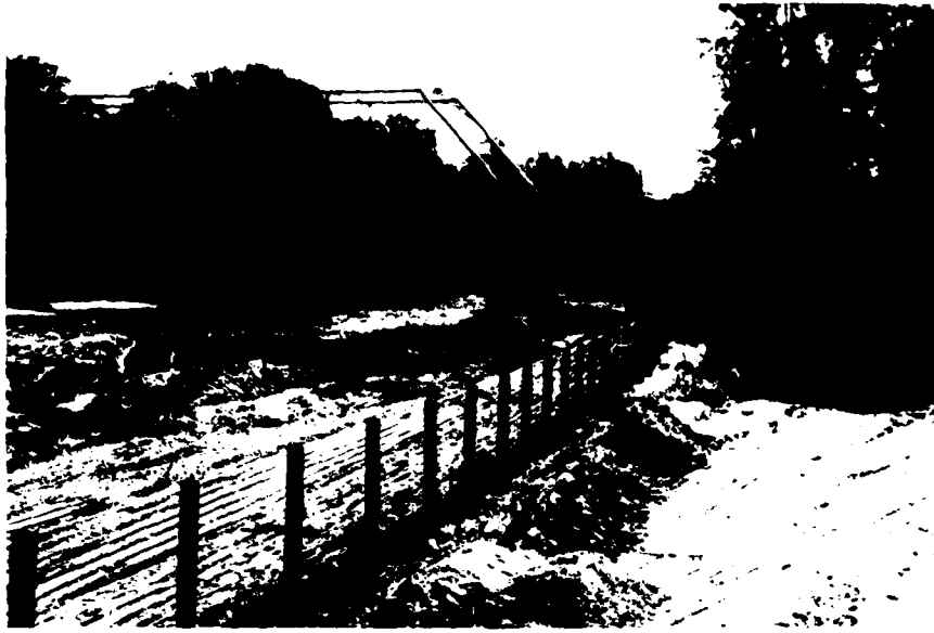
a. Downstream view of wire fence revetment. Schroyer Bridge is in the background
