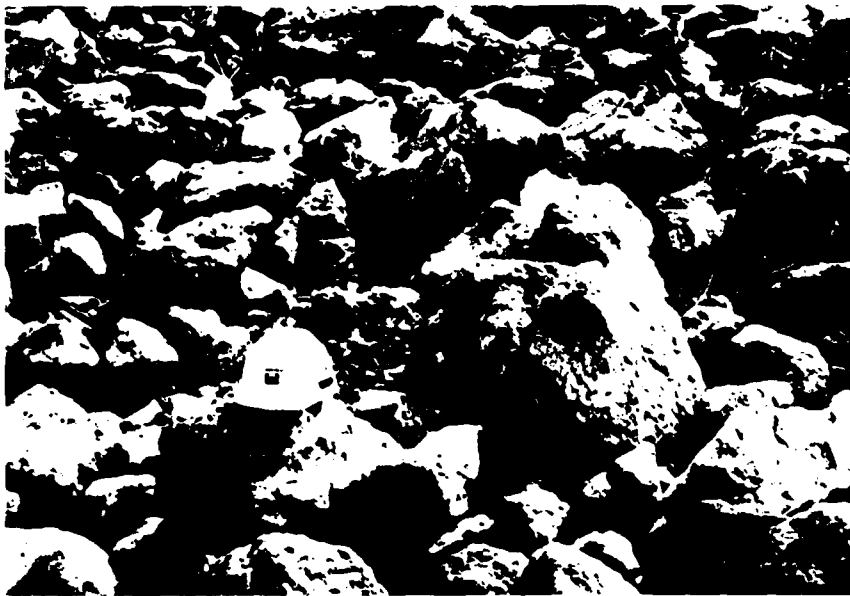
Figure 27. Republican River at Milford Dam Outlet Channel, Kans. The area behind the hard hat is typical of the isolated areas of exposed bedding material in Test Sections 1 and 2 (May 1977). (Source: Reference 11)
