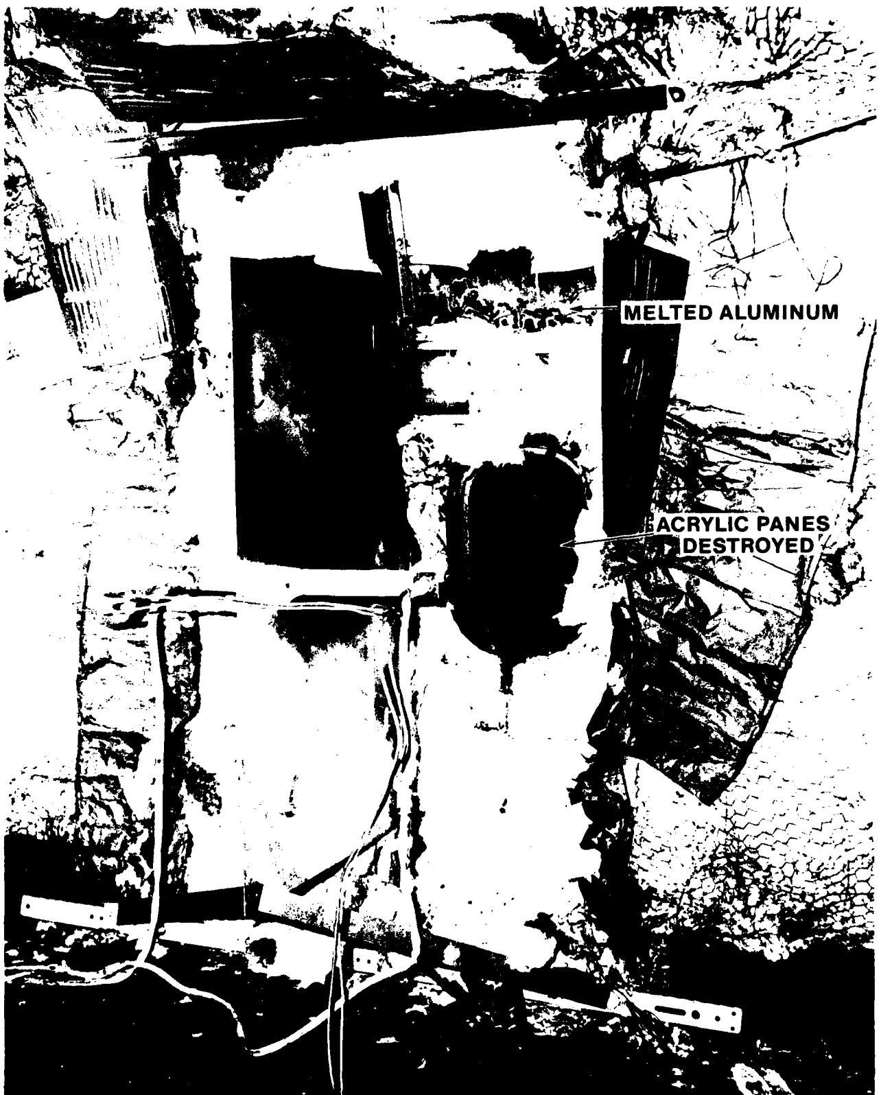
FIGURE 9. FIRE DAMAGE TO THE STANDARD DC-10 WINDOW SYSTEM SHOWING THE COMPLETE DESTRUCTION OF THE ACRYLIC WINDOW PANES (TEST 1)
