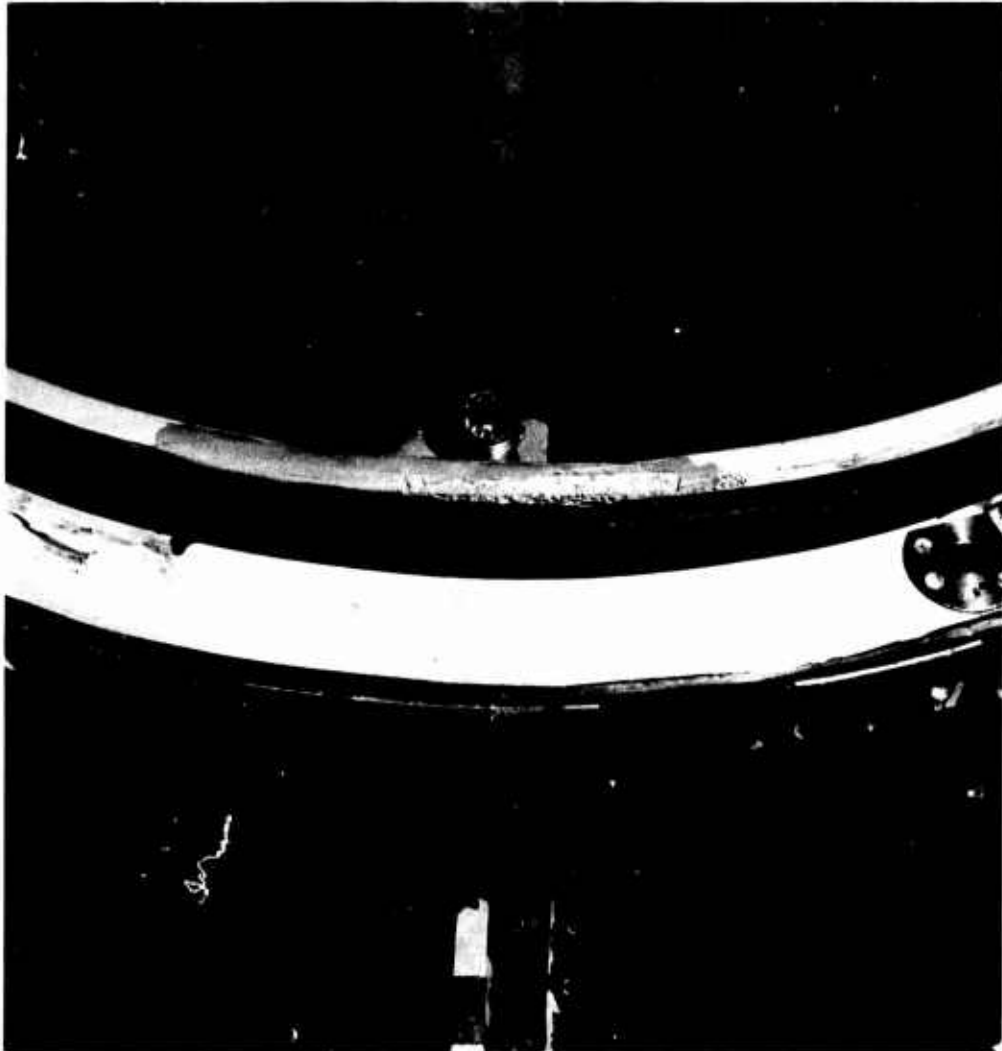
Figure 9. Corrosion of a metal surface which had been exposed to a porous moistured material
