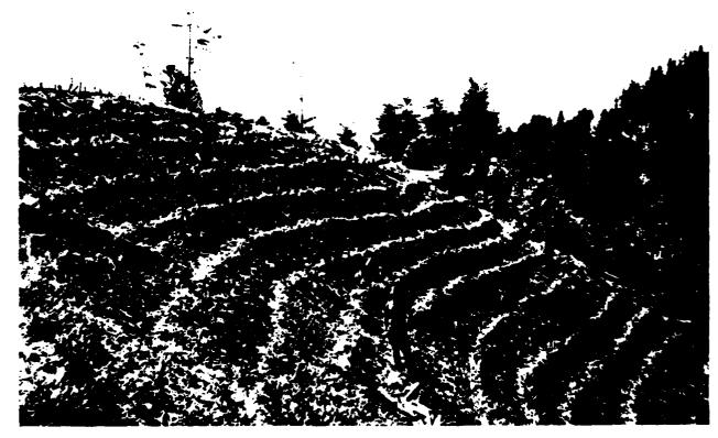
Fig. 2.7Slope protected by contour-wattling. Partially buried and staked willow wattles protect slope against erosion; wattles eventually root and sprout, thus further stabilizing the slope. Redwood National Park, California.
