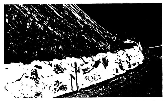
Fig. 2. 14 Breast wall defense at toe of slope adjacent to roadway. Contour wattling and slope plantings are visible through holdown netting used on face of slope.
