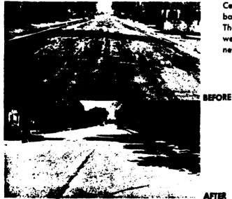
Cement treated base solved the problem of rebuilding failed flexible base streets in the Bel Air residential subdivision at a minimum cost. The existing base material and some of the worn out asphalt surface were salvaged, mixed with portland cement and water to provide new durable CTB streets.
