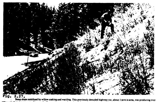
Steep slope stabilized by willow staking and wattling. This previously denuded highway cut, about 1 acre in area, was producing over 100 cu yd of erosion per year. Unrooted willow cuttings were planted on 2-ft centers, and about 1100 lineal ft of willow wattling were also installed. The stuck cuttings and willow wattles have rooted and sprouted vigorously as shown. Erosion and bank sloughing problems have been virtually eliminated at this site. State Highway #89, near Luther Pass, California.
