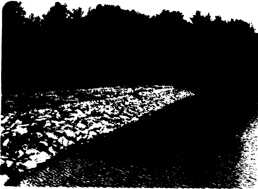
PHOTO #7: Riprap on Upstream Face of Dam, looking West from Intake Structure.
