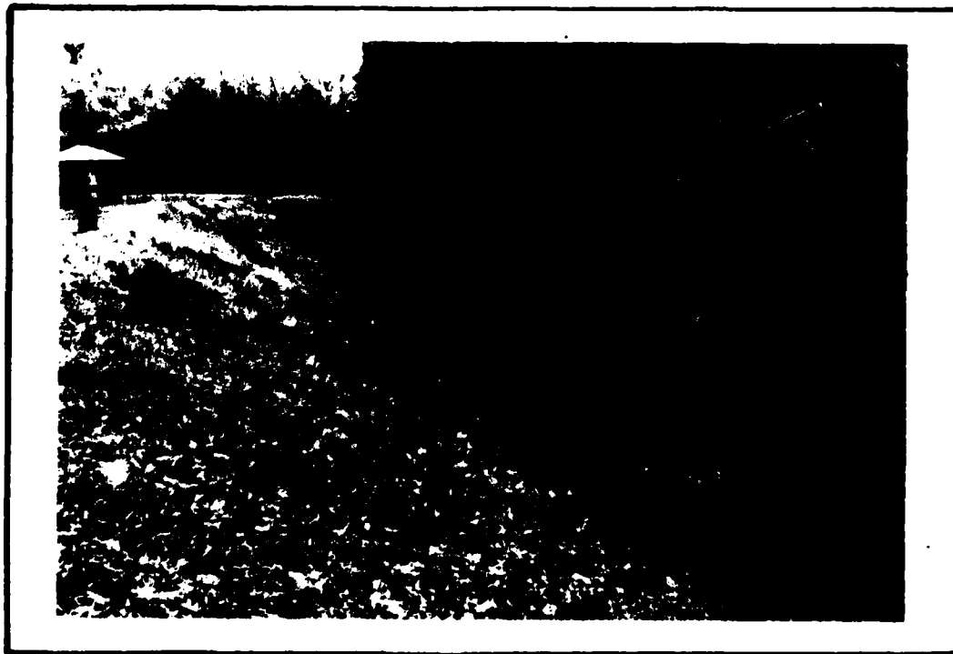
4. DOWNSTREAM FACE OF THE DAM SHOWING SIZEABLE TREES GROWING ON THE EMBANKMENT. (11/13/79)
